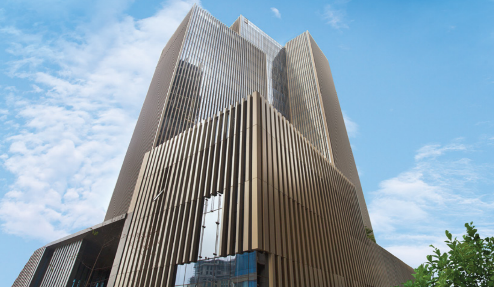
ALUCORE® | Max Towers – Noida, India Architect: Gensler | Fabricator: Ashbee Industries India Pvt. Ltd. Photography: © Rohit Kumar
