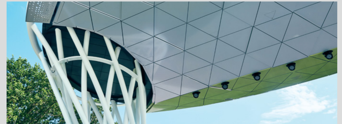
ALUCOBOND® PLUS | Lauridsen Amphitheater, Des Moines, USA Architect : RDG Planning & Design | Fabricator : Metal Design System Inc.; The Waldinger Corp. Photography: © Joe Crimmings
